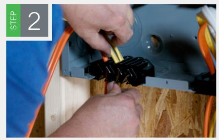
Slide the wire into the slot
